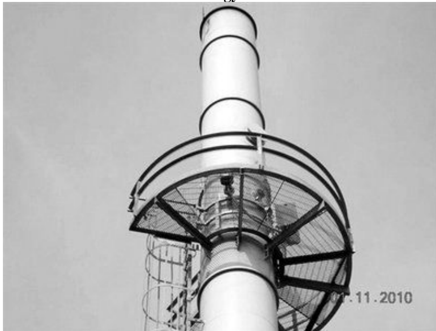
Smokestack of a Waste to Energy Biomass Gasification Plant 1
