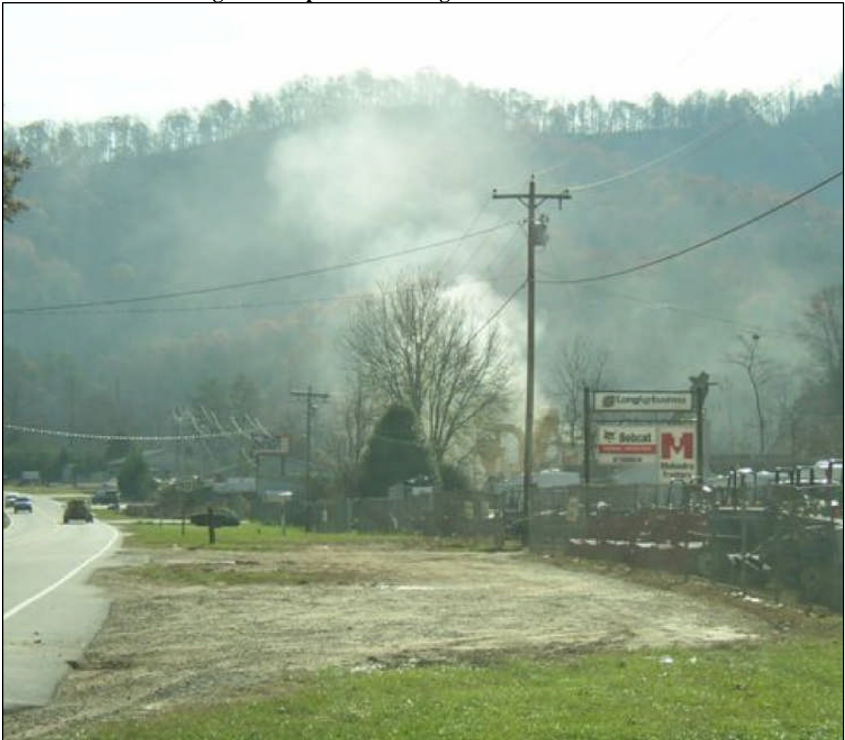
Figure 1. Asphalt Plant Fugitive Emissions
